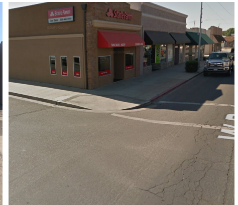
Curb ramp does not align with crosswalk at intersection of Robertson Boulevard/3rd Street.
