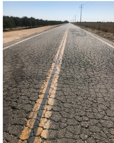
Alligator Cracking on Avenue 26 near Road 19
